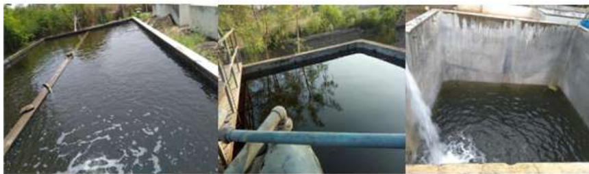
Storage Tanks for Treated Water (Before Reuse in the Garden)
