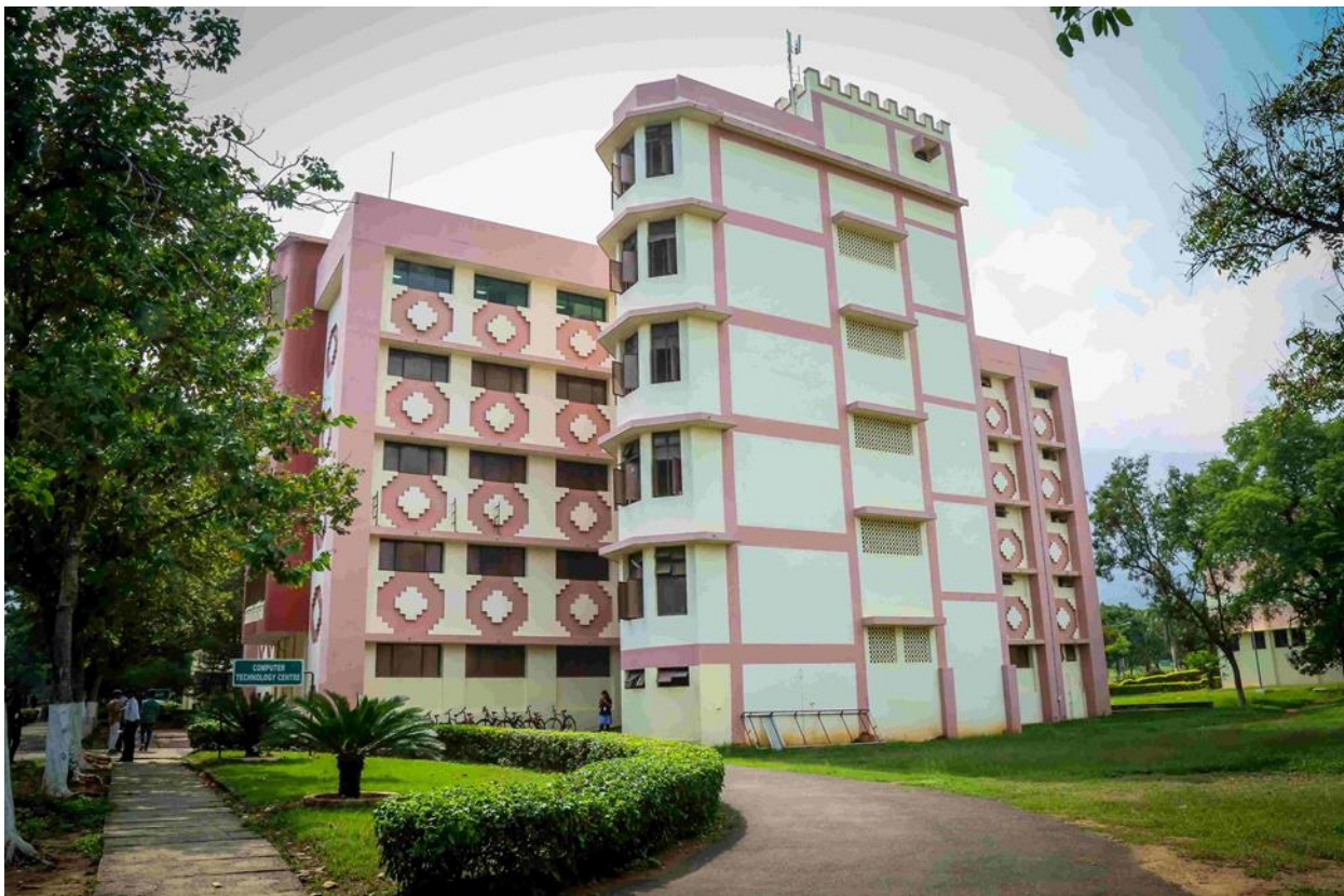
Computer Technology Centre
